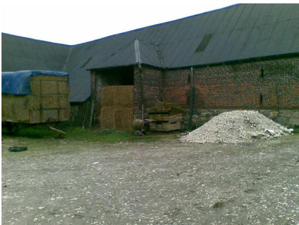
**Figure 5.3** Historic farm buildings may have potential for wood chip production. With a concrete floor this barn could be used for chip storage and the yard for timber storage and seasoning before chipping. Limited ventilation might prove problematic with this building if the chip is not thoroughly air dried.
